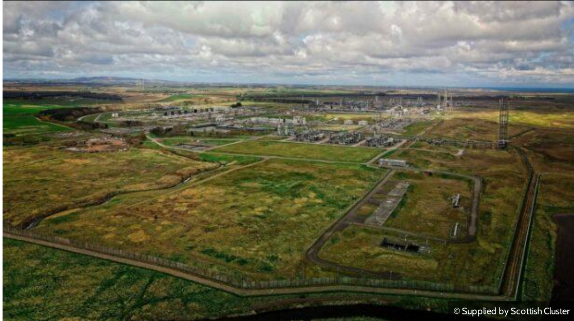
The St Fergus gas terminal which houses Storegga's Acorn project
